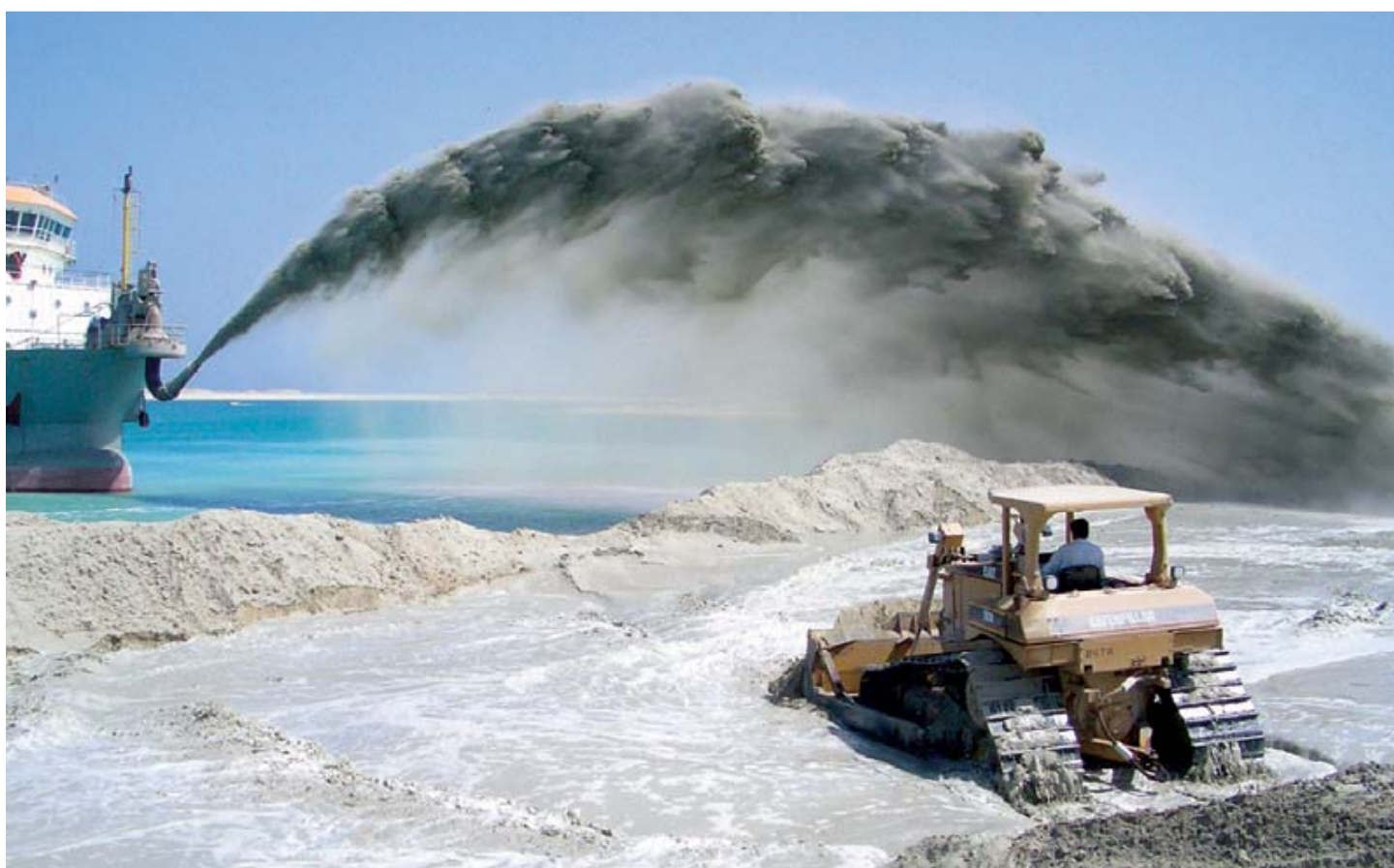
Trailing Suction Hopper Dredge rainbowing sand.
